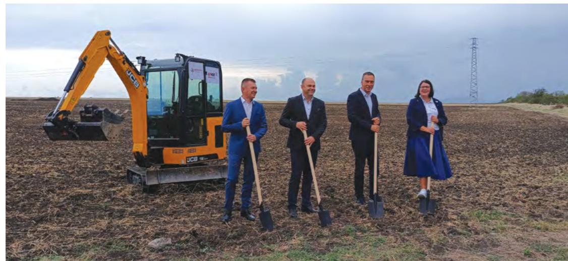
The construction works for underground laying of the overhead power lines with a total length of 20 kilometres were launched at a ceremony on 28 September 2023 by Eng. Stoycho Valchev, Executive Member of the Board of Directors of EP Yug, Eng. Zdravko Bratov, Deputy Chairman of the Board of Directors of EP Yug, Dimitar Nikolov, Mayor of Burgas Municipality and Vanya Ratarova-Georgieva, Executive Director of BSPB (pictured left to right).
